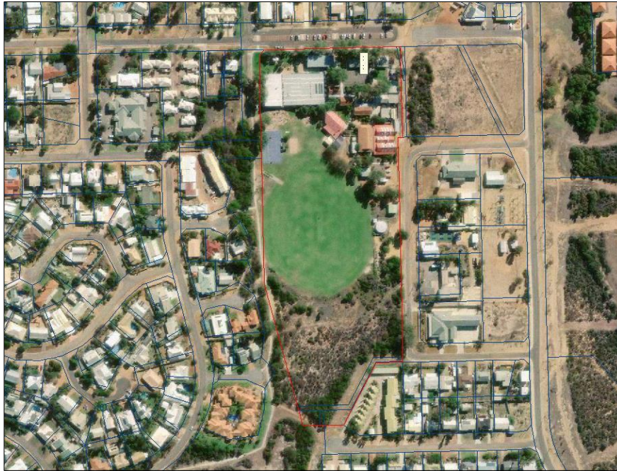
Figure 2. Site plan of location of Virtual Power Plant at Kalbarri District High School
