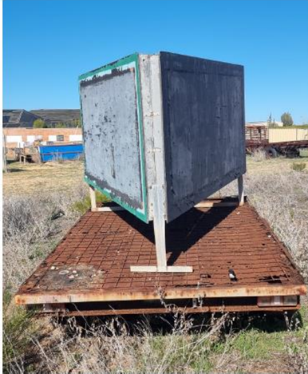
Existing sign to be refurbished and relocated to new trailer.
