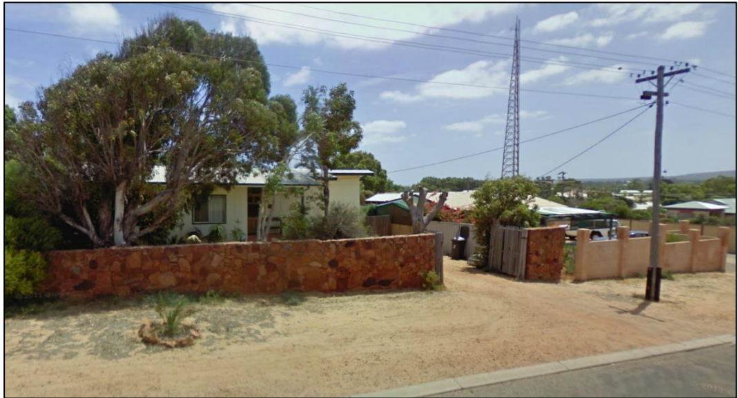
Figure 2. – View looking north towards Lot 179 (No.13) Glass Street, Kalbarri
