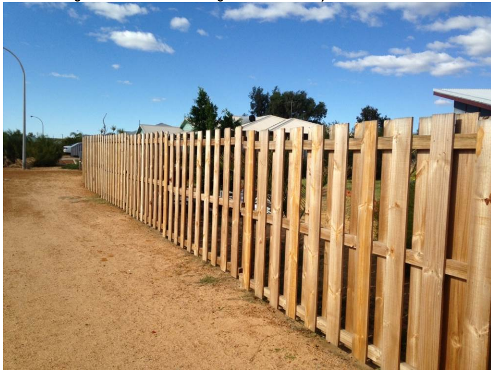
Below: 1.8m high fence erected along front boundary to be stained cedar in colour
