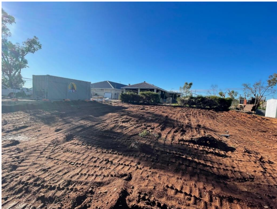
Western side of site up to school
