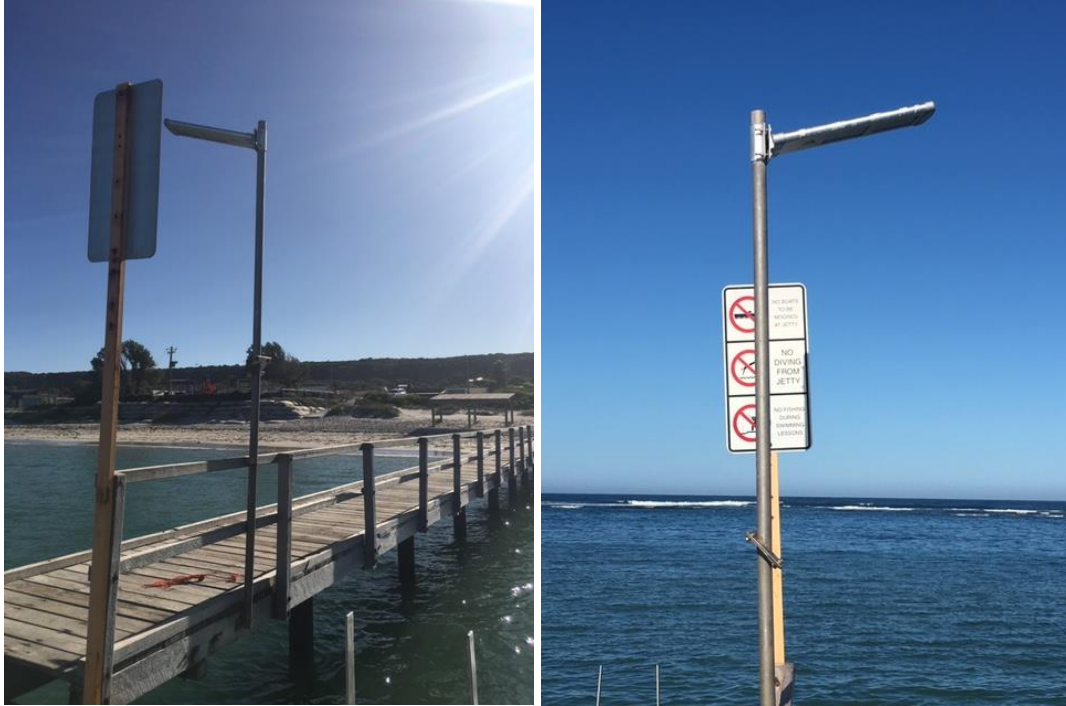
New light at end of jetty
