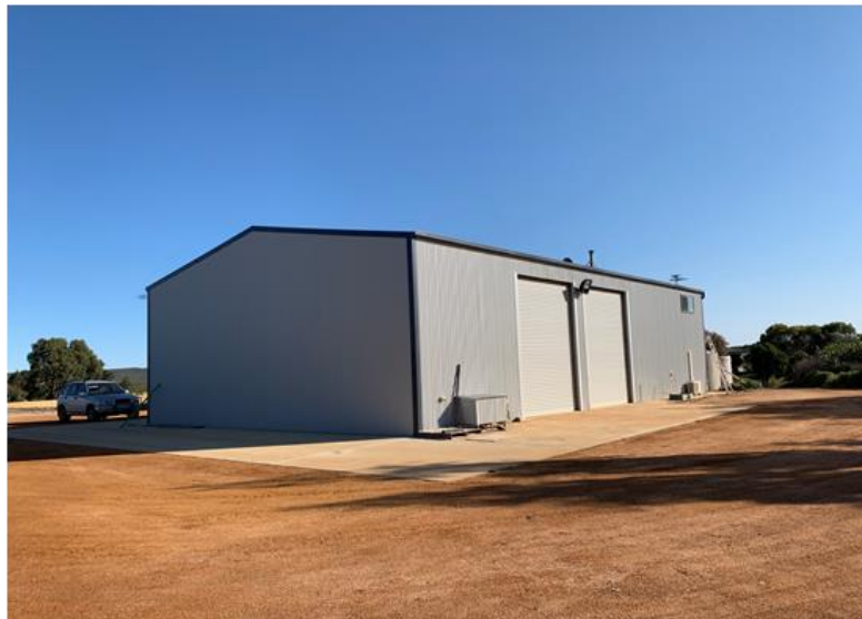
Western and southern elevations
