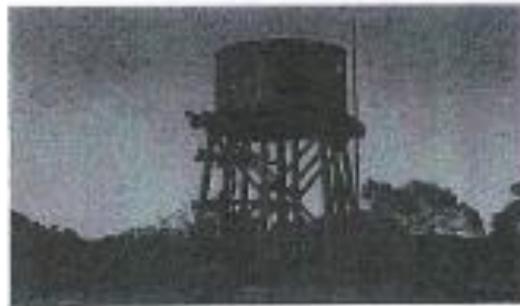
View of the Railway Tank on the Ajana Back Road
