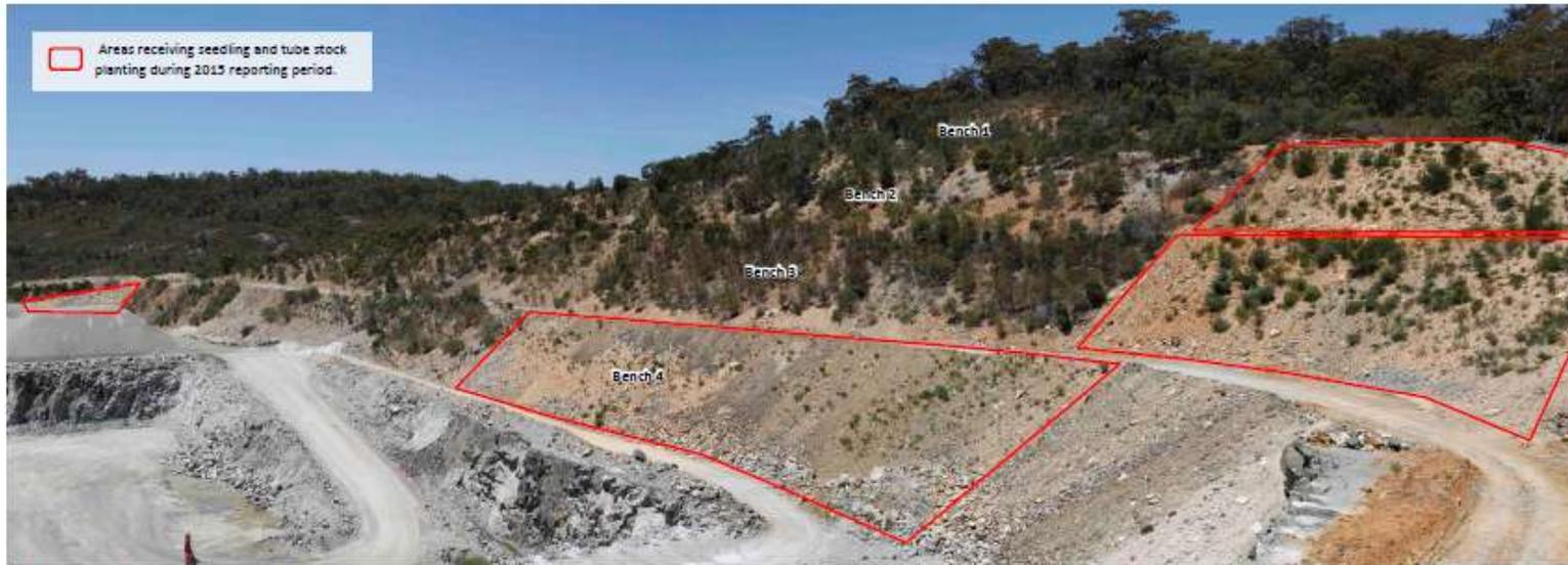
Photo 9: Rehabilitation eastern face of Stage 3 Pit.
