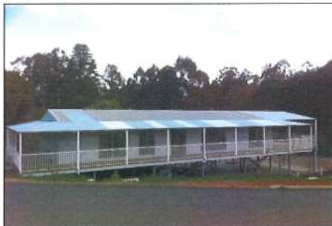
Example transportable being refurbished Shire of Bridgetown-Greenbushes
