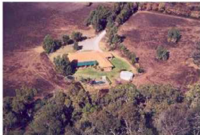
Reduced fuel in the Building Protection Zone contributed to the survival of this home in a bushfire.
