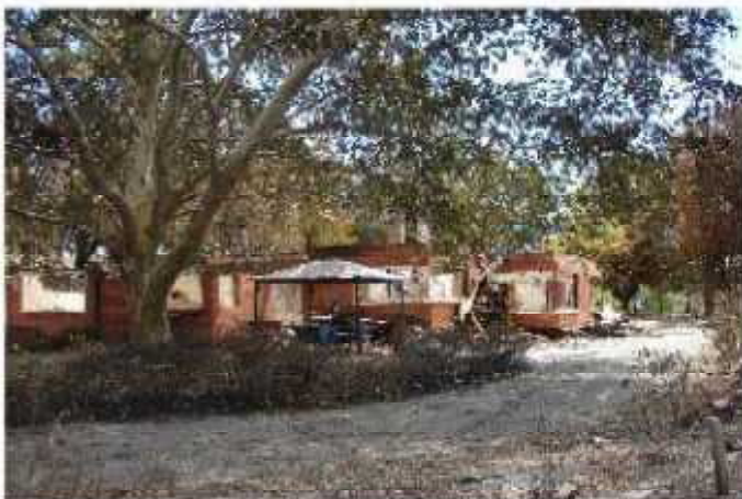
A home destroyed by bushfire, note the tree branches overhanging the house.
