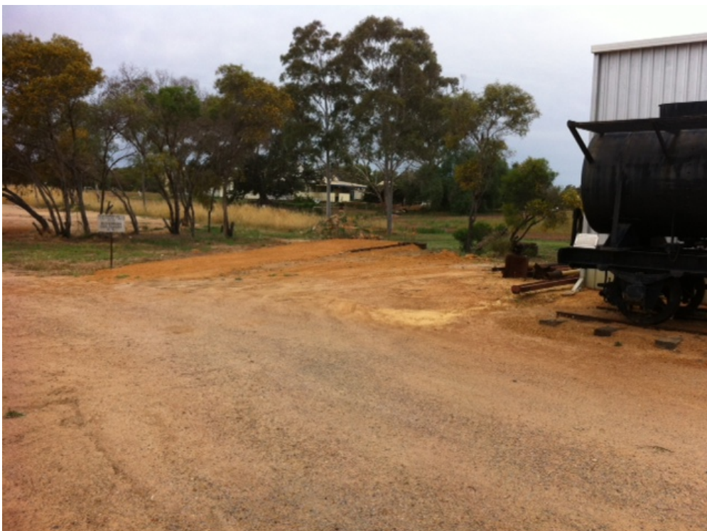
Gravel pad for carriage site
