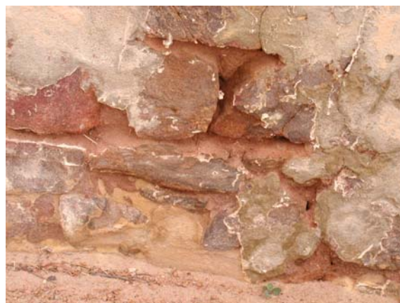
The colour of the deteriorating render suggests that cement has been used in past repair works.
