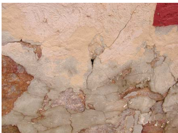
Beneath this section of render there has been substantial deterioration of the stone.
