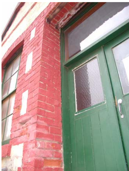
Deterioration to brickwork to entry door reveals
