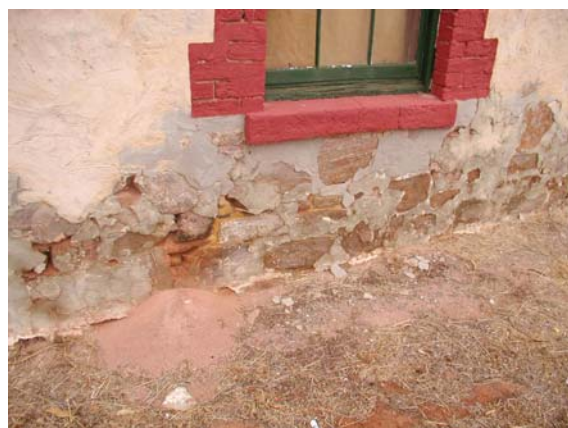
Beneath this section of render there has been substantial deterioration of the stone.
