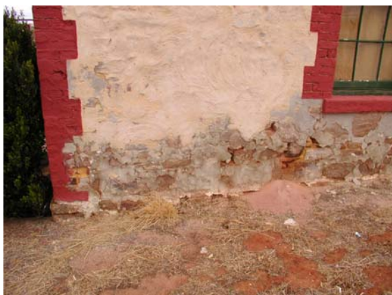
The colour of the deteriorating render suggests that cement has been used in past repair works.
